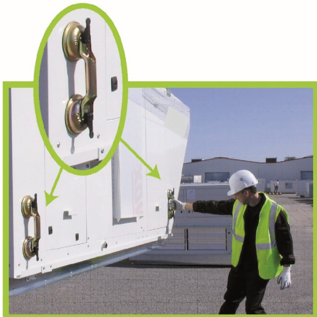
Vacuum lifting beam to position the unit
