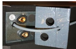
The pre-cut insulation foam is easy to fit and guarantees total isolation of the casing once all tubes have been connected.
