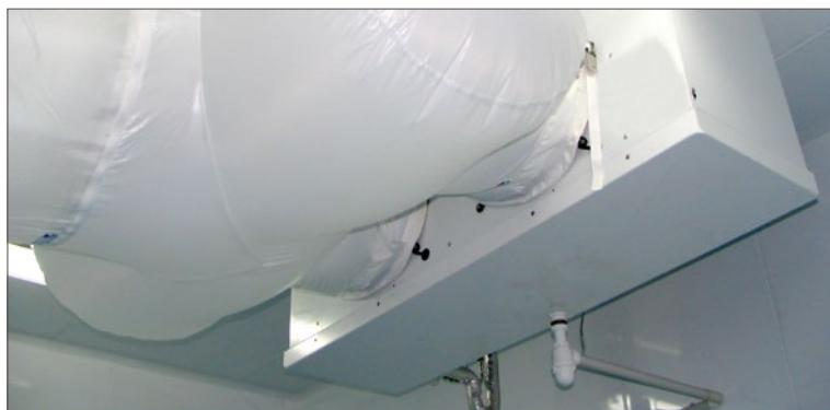
**VGT option** used to fasten the textile duct (not supplied).
