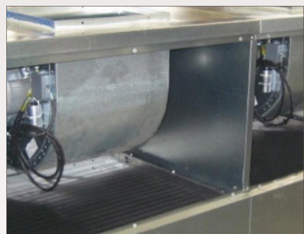
In order to facilitate pressure control with fan stoppage, the turbines are separated with a baffle to avoid air by-pass.
