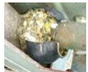
Galvanic corrosion under the plastic sleeve.
