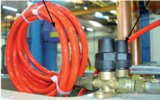
High pressure Lines ready to be connected to the valve Refrigerant shut off valve
