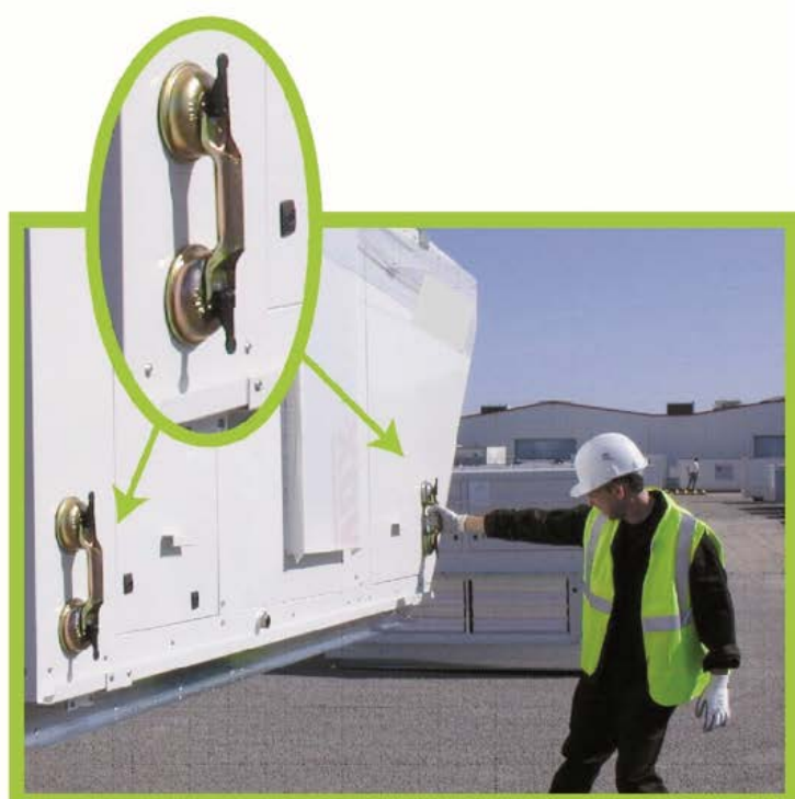
Vacuum lifting beam to position the unit
